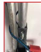
Drill Hole through Lid and upper tent pole attach with fender washers and bolt use zip-ties below bolt, you may have to notch the lid to get the pole to set flush.
